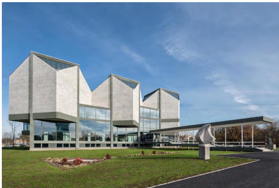
Figure 17 The exterior of the Museum of Contemporary Art in Belgrade, after the reconstruction, 2017
