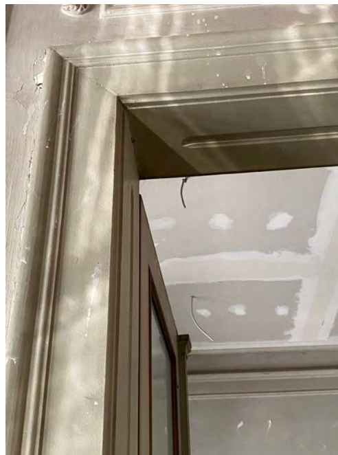
Fig.17. Execution of plaster work
