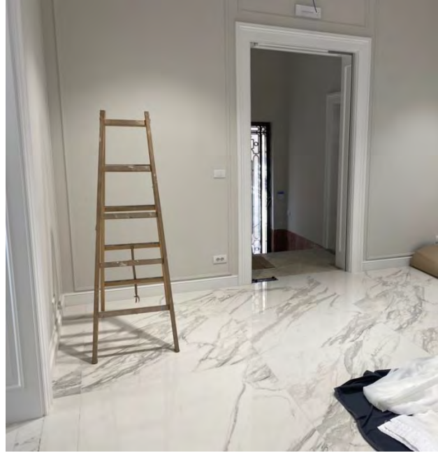
Fig.19. Final interior works
