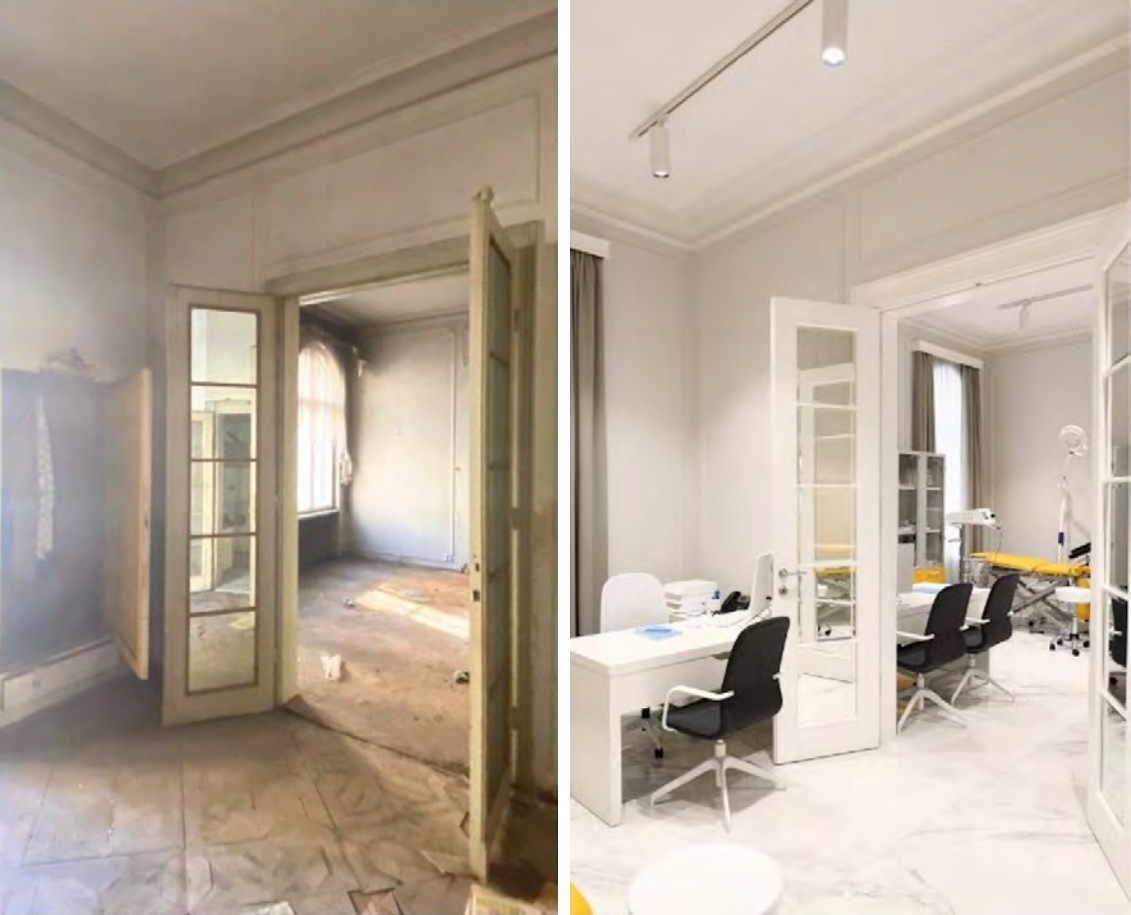
Fig.20,21. Photographs of the examination room before and after adaptation
