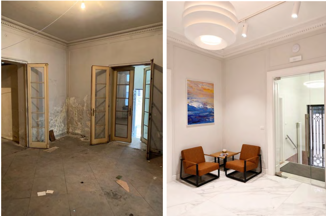
Fig.24,25. Photographs of the entrance hall before and after adaptation
