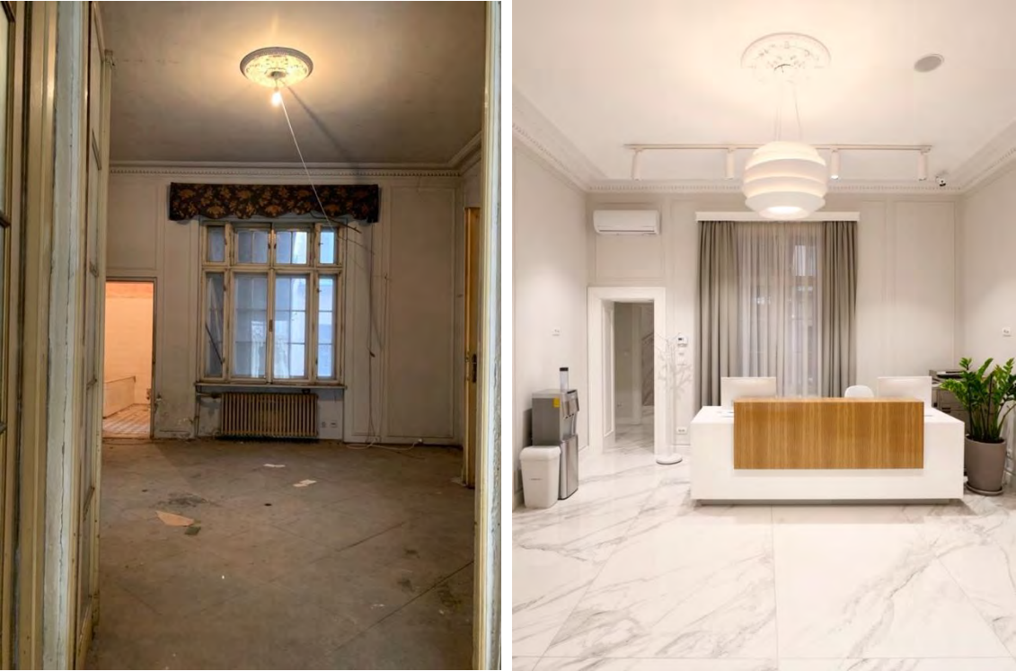
Fig.22,23. Photographs of the entrance hall before and after adaptation
