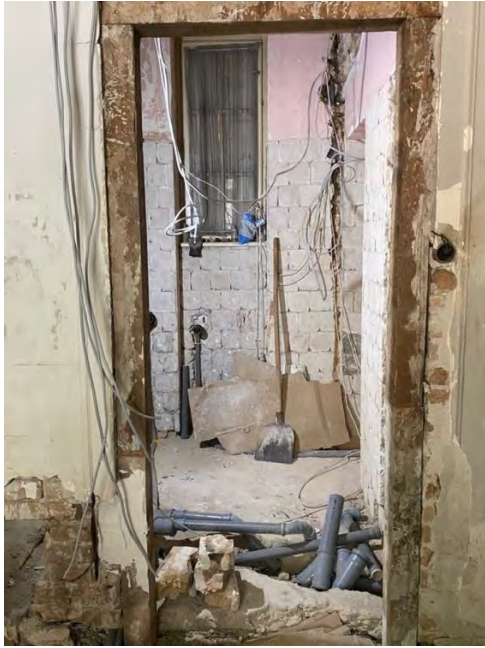
Fig.18. Replacement of electrical installations
