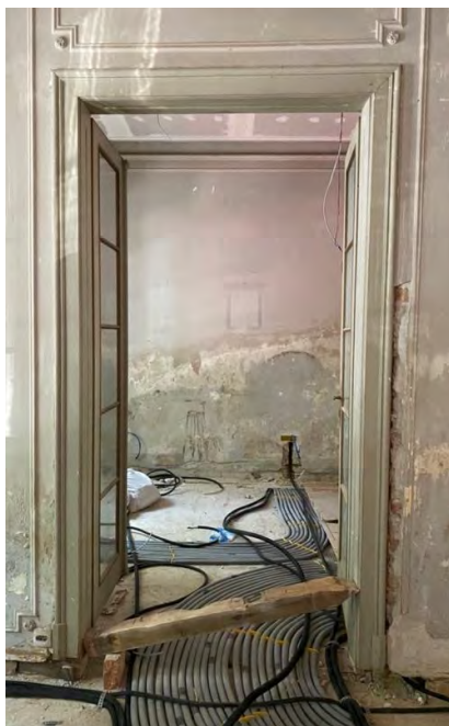
Fig.16. Installation of underfloor heating
