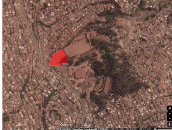
Figure 22 A site location for the Ebola Treatment and Community Center
