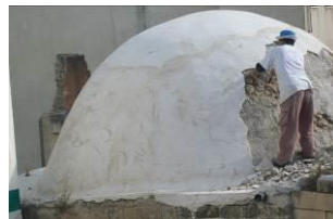
Figure 12: Removing cement plaster from the outer surface of the dome.
