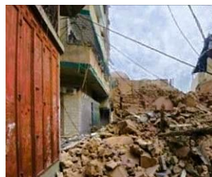
Figure 16: destruction of the southern and northern parts of the house
