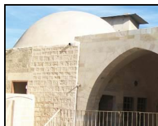
Figure 13: First floor domed room and iwan after conservation.
