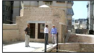
Figure 5: First floor cross vaulted room after renovation, Dr. Abdurrahman Mohamed (middle) and ICRC economic security commissioner, Jerusalem office (right).
