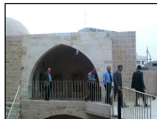
Figure 4: First floor iwan after renovation.
