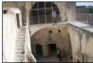
Figure 8: East elevation of the courtyard before preservation
