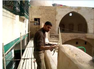
Figure 9: Outdoor plaster works.
